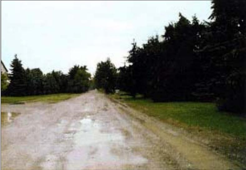
Applying a Double Chip Seal Surface will eliminate the need for grading and dust control. If your base is not sufficient, we will add base material and grade your existing road to ensure proper drainage. Ditches and drains that work are most important for making any new road surface work. The picture at left shows the road condition of Dinsler Road in Novi before our preparation.
